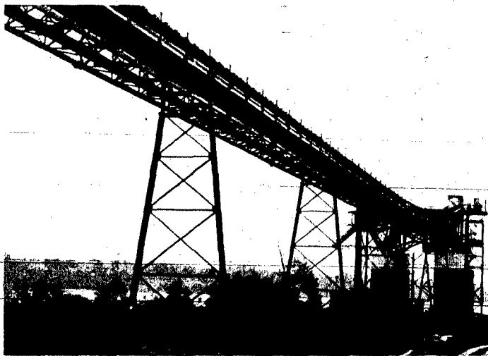
This coal-carrying belt, 6 miles in length, is the latest method of materials handling in the Midwest coal belt.
